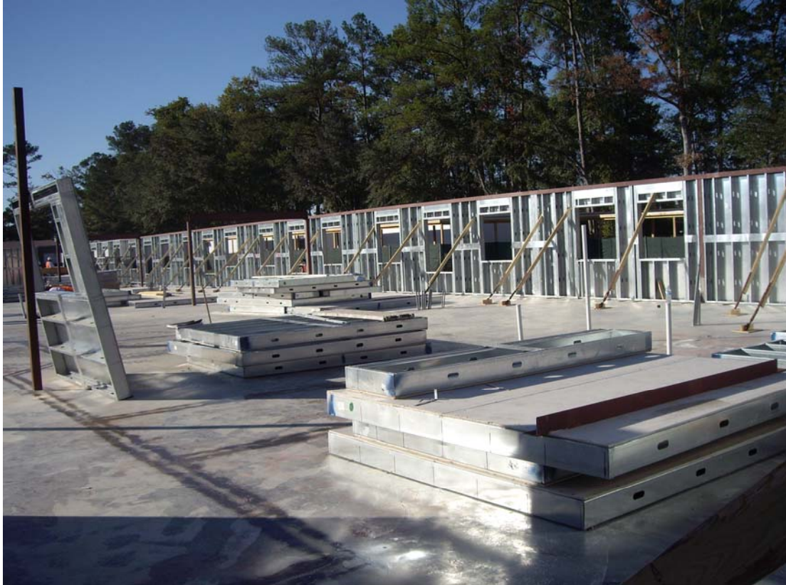
Exterior and interior load-bearing 'Sure-Board Wall Panels' are quickly and easily erected.
