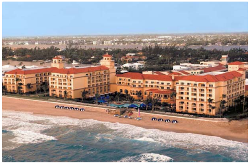
The Ritz-Carlton, Location: PALM BEACH, FL Project: Spa Expansion Completion: March 2009
