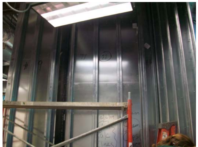
Sure-Board installed on interior steel stud walls designed for Blast resistance
