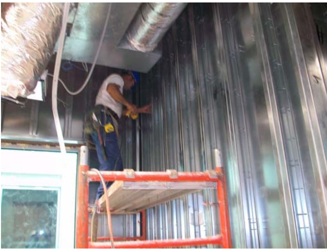
Sure-Board installed on interior steel stud walls designed for Blast resistance
