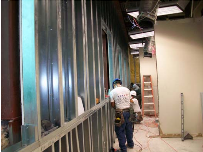
Sure-Board installed on interior steel stud walls designed for Blast resistance
